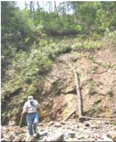
Photograph 8.3 Mass landslide on the Pachum riverbank, north of the project area
